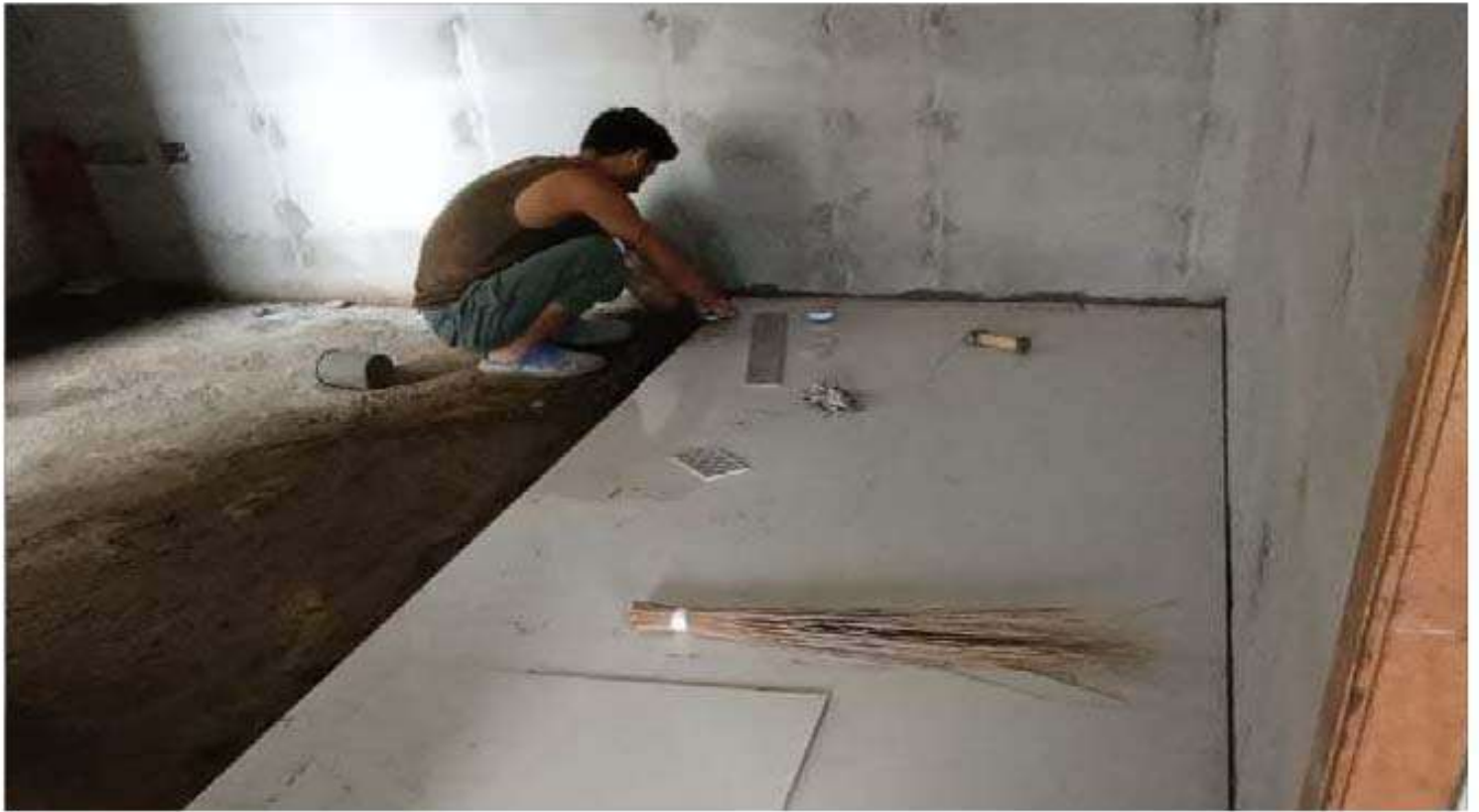
BLOCK 2 FLOOR TILES WORK IN PROGRESS
