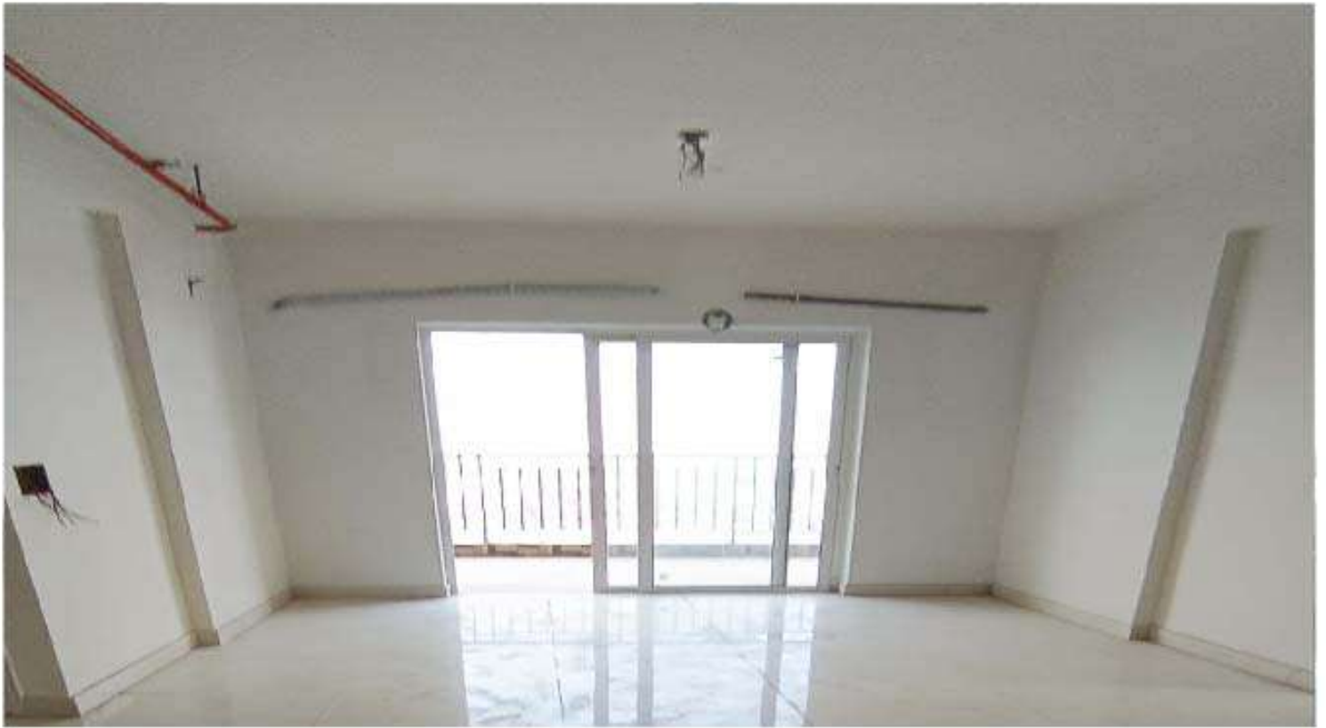
BLOCK 3 - FLOORING COMPLETED
