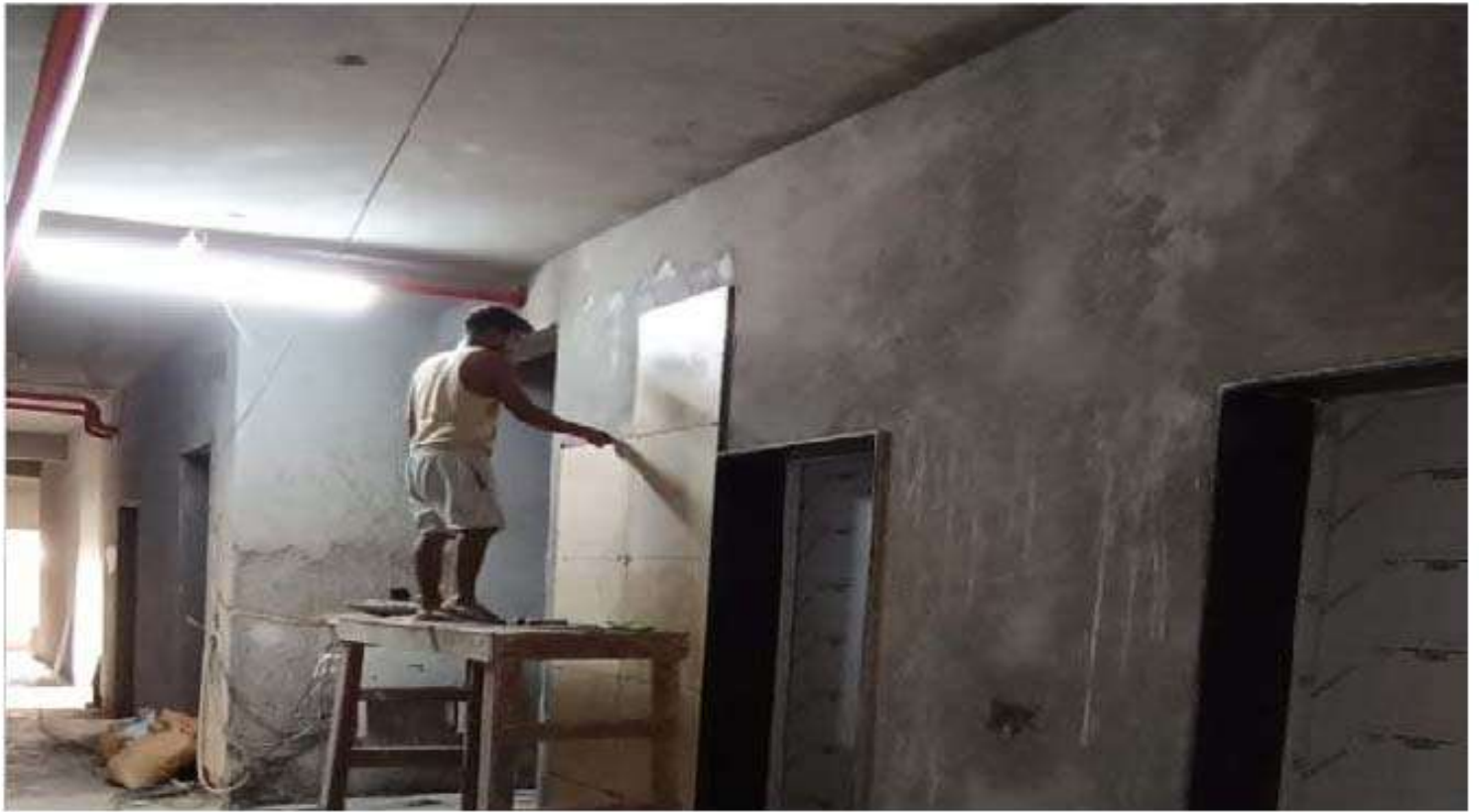
BLOCK 2 - LIFT LOBBY AREA TILES WORK IN PROGRESS
